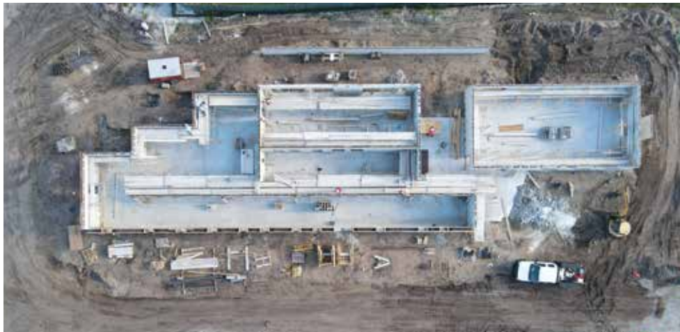
WALLS GOING UP
