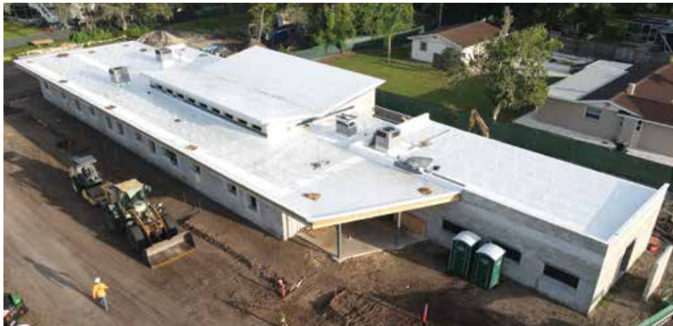
FINISHING UP ROOF
