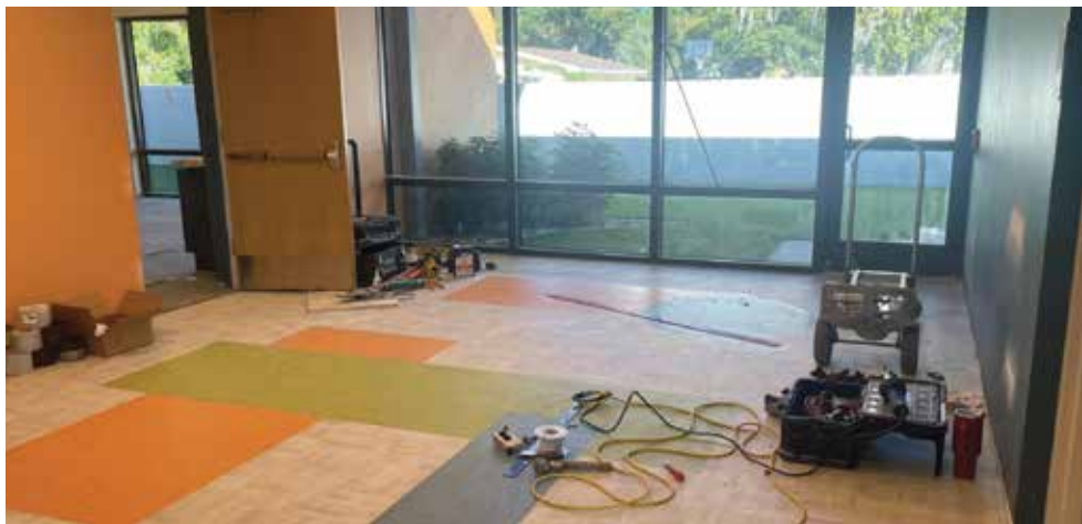
INTERIOR COMING TOGETHER
