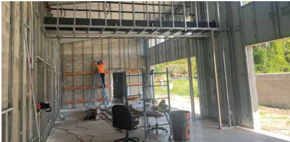
FRAMING OUT INTERIOR
