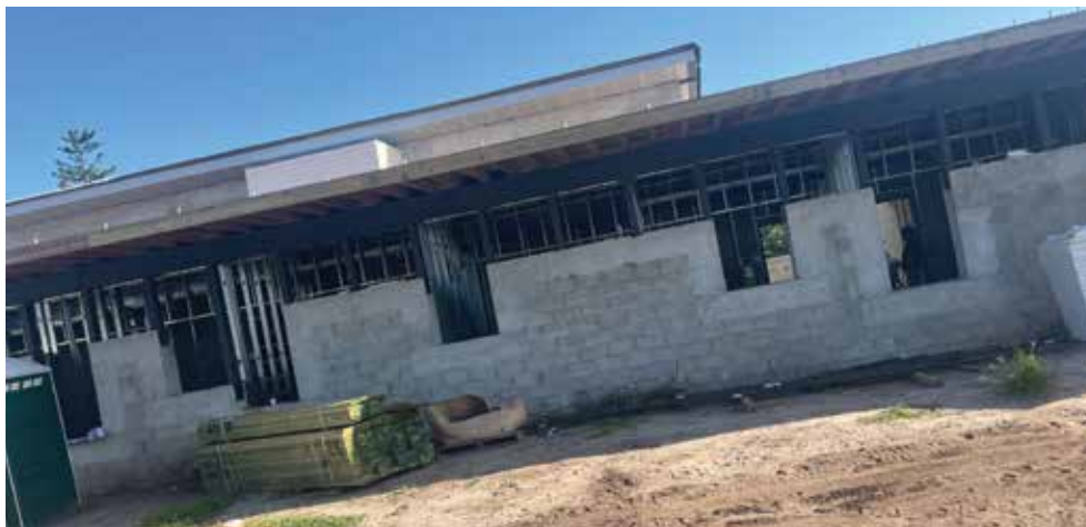
ROOF GOING ON
